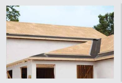
Water & Ice Protection is a 55-mil flexible rubberized asphalt, fiberglass-reinforced membrane used as a shingle underlayment on critical roof areas such as eaves, ridges, valleys, dormers and skylights. Water & Ice Protection underlayment protects roofing structures and interior spaces from water penetration caused by wind-driven rain and ice dams and may also be used as covering for the entire roof to prevent moisture or water entry.
